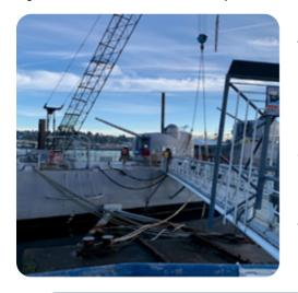
protecting Bremerton Marina, we in turn assist with their upkeep. Recently, the Turner Joy needed maintenance on their gangway and related mechanisms. A floating crane was utilized to repair the mechanisms that allow the gangway to move and flex with the tides twice each day. Port staff assisted the nonprofit with the provision of welding equipment and general project support, and while the museum was closed for two weeks during this project, they are now reopened with regular hours.
